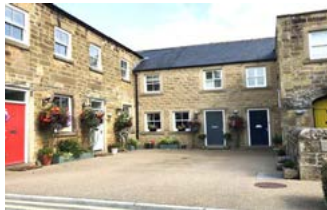
Individual painted doors in courtyard
